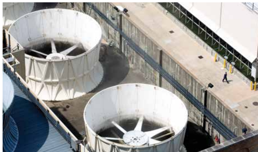
A TECO employee walks the roof of the plant. Massive fans help cool chillers that are used to generate chilled water and keep temperatures comfortable in more than 20.3 million square feet of building space on the TMC campus.
